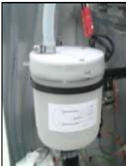
Floating water level detection device
